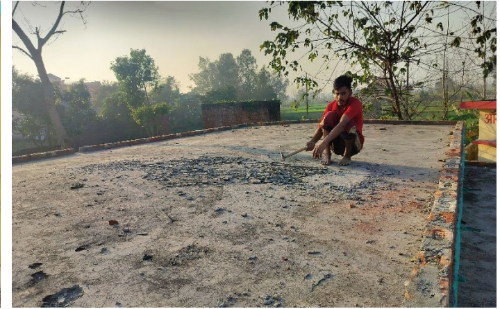
Main building water proofing
