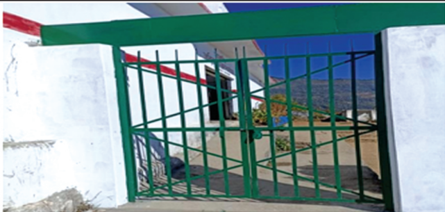
School Gate Repair
