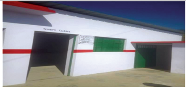
Complete school work with white wash window work After
